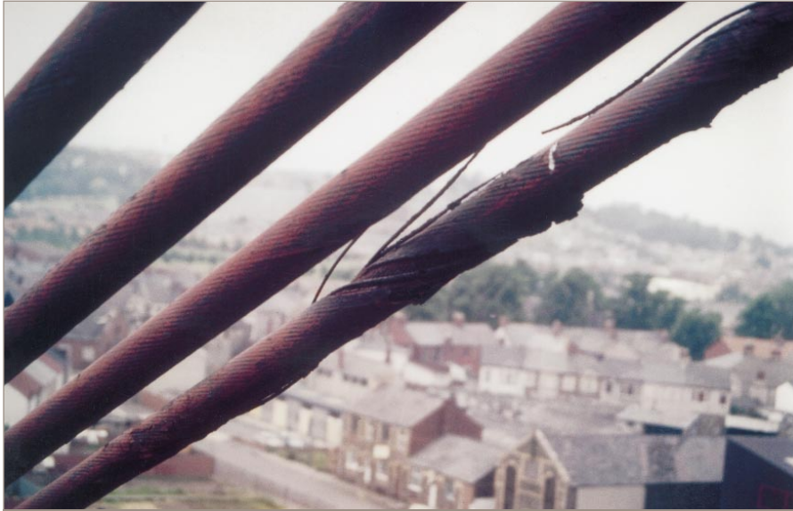
Fig. 6. Main cable wire breakages
